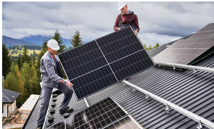
Workers install solar panels on the roof of a house.
