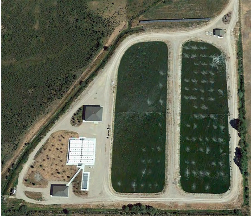
The Driggs wastewater treatment plant is an example of a larger lagoon system with some additional technical aspects. / Google Earth
