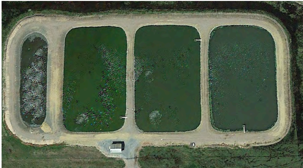
The Inkom wastewater treatment plant is an example of a small lagoon-based facility. / Google Earth
