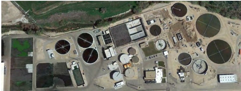
The Nampa wastewater treatment plant is an example of a large facility with mechanical and biological treatment. / Google Earth
